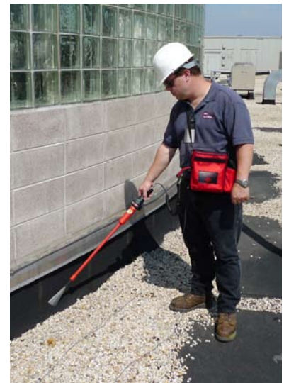
High voltage vector mapping (dry testing) is ideal for testing flashings and other vertical surfaces.
