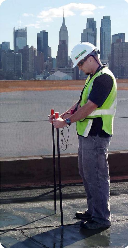
In Low Voltage Vector Mapping (wet testing) the technician uses metal probes on a wet surface to pinpoint membrane breaches.
